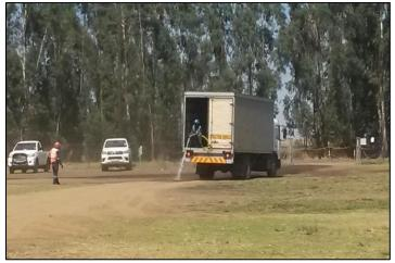
Figure 2: Spraying water for dust control.
