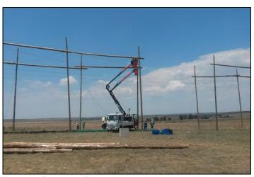
Figure 3: Erecting of H- poles.
