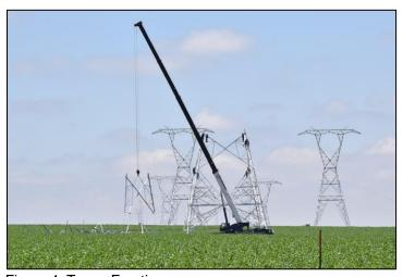
Figure 4: Tower Erecting.
